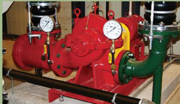
East Hartford High School —EnviroFlo Horizontal Split Case Pumps met critical construction schedule demands with easy, groutless base installation. Now they're providing high efficiency primary/secondary chilled water and condenser water movement for reliable student/teacher comfort.
